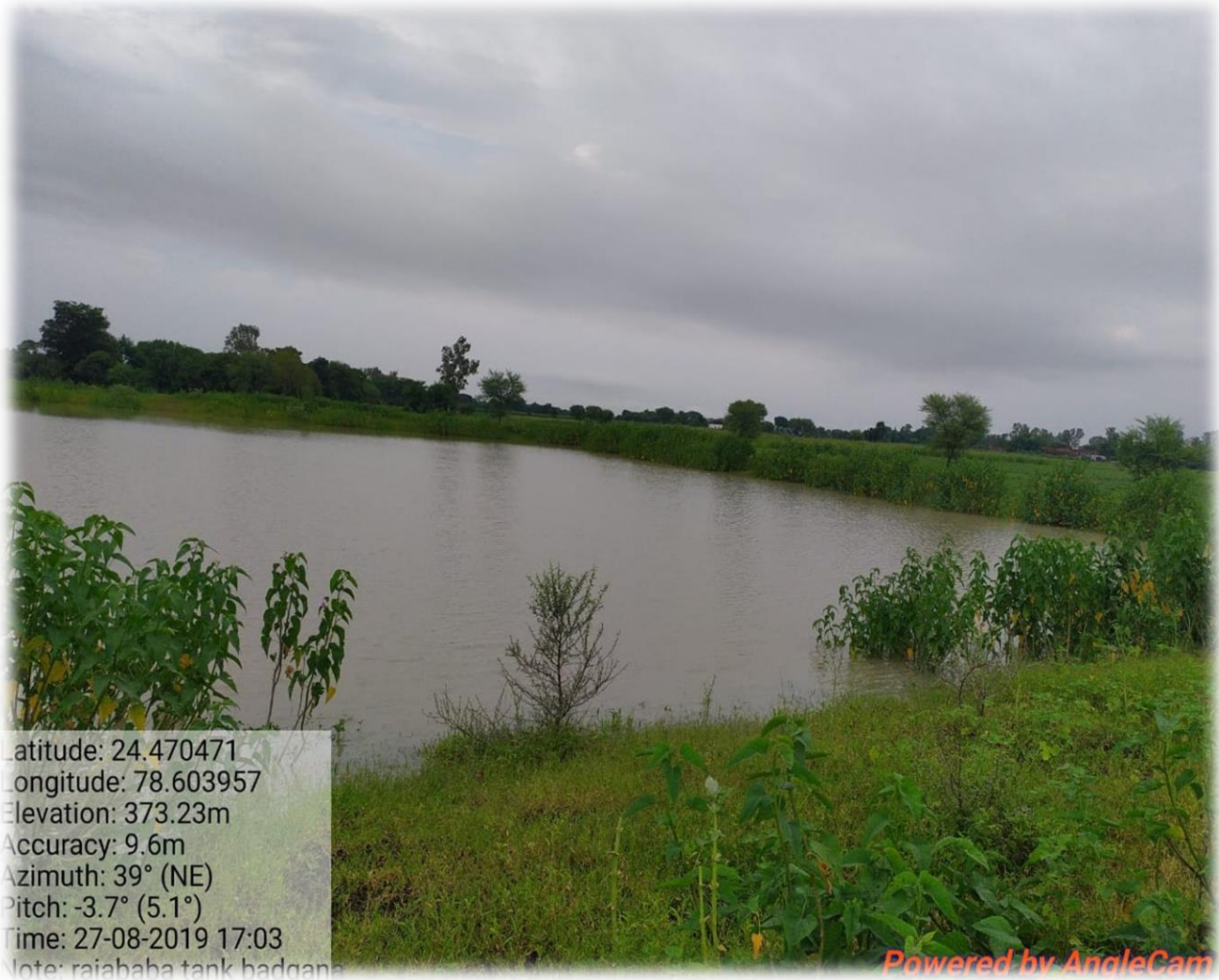
Photo of Raja Baba Tank Village Badgana , Filled with rain water After De-Siltation Work.
