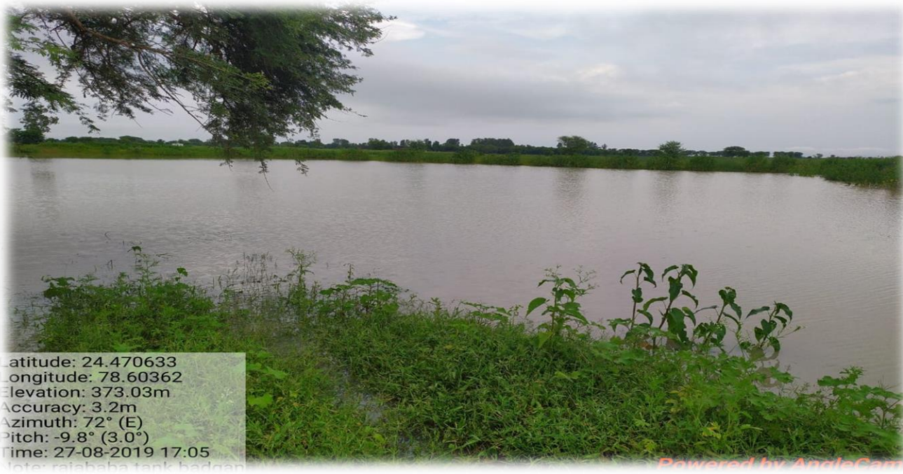
Photo of Raja Baba Tank Village Badgana , Filled with rain water After De-Siltation Work.
