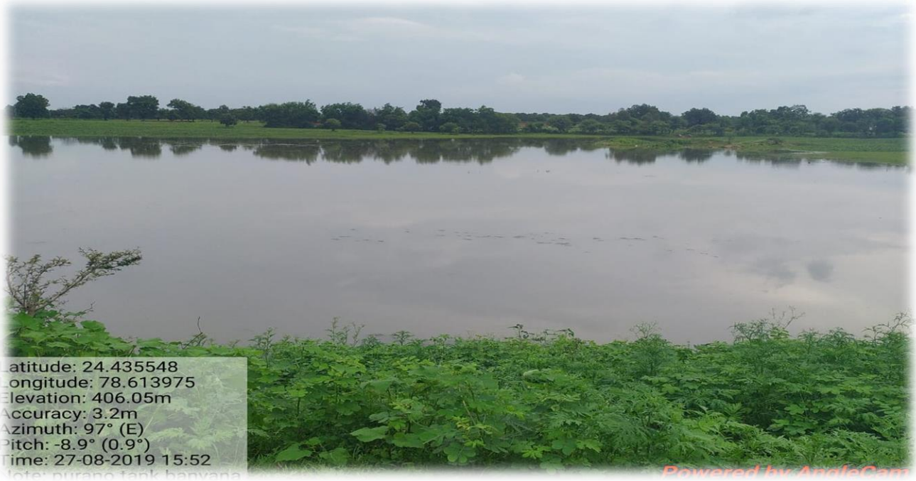
Photo Of Purano Tal Tank Village Banyana , Filled with Rain Water After De-Siltation work .
