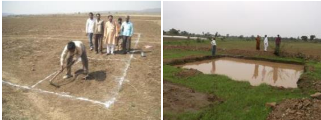
(Left) Demarcation of a pond on the field of a farmer and (right) pond filled with water
